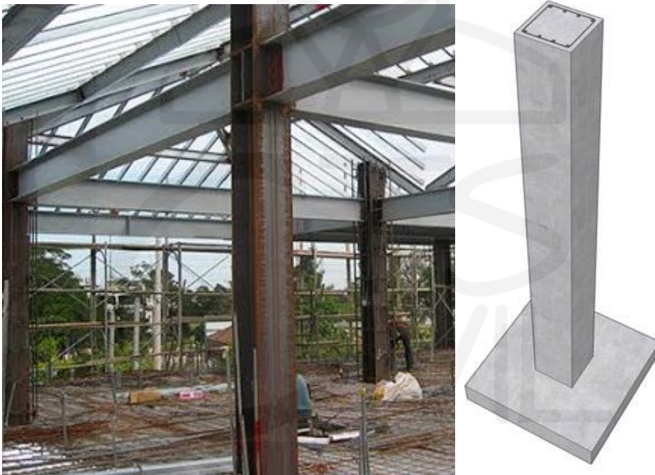
Figure 1-4: Steel and concrete columns
