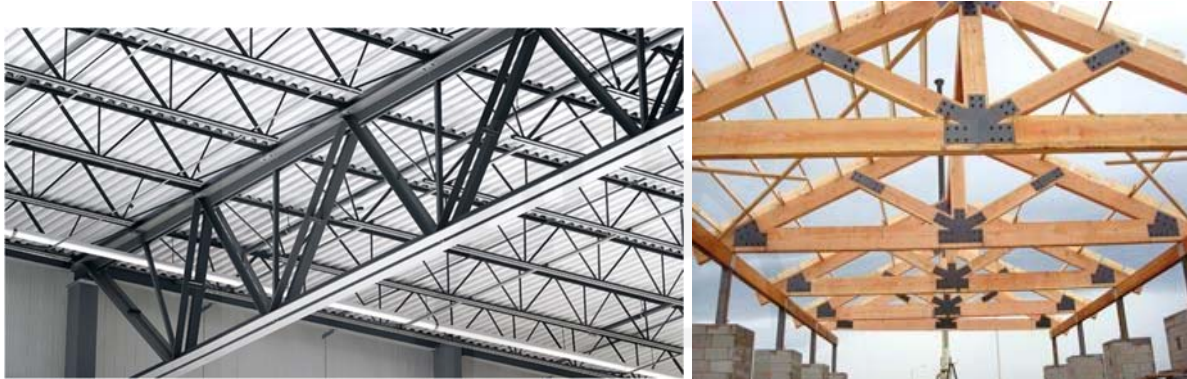
Figure 1-5: Steel and timber trusses
