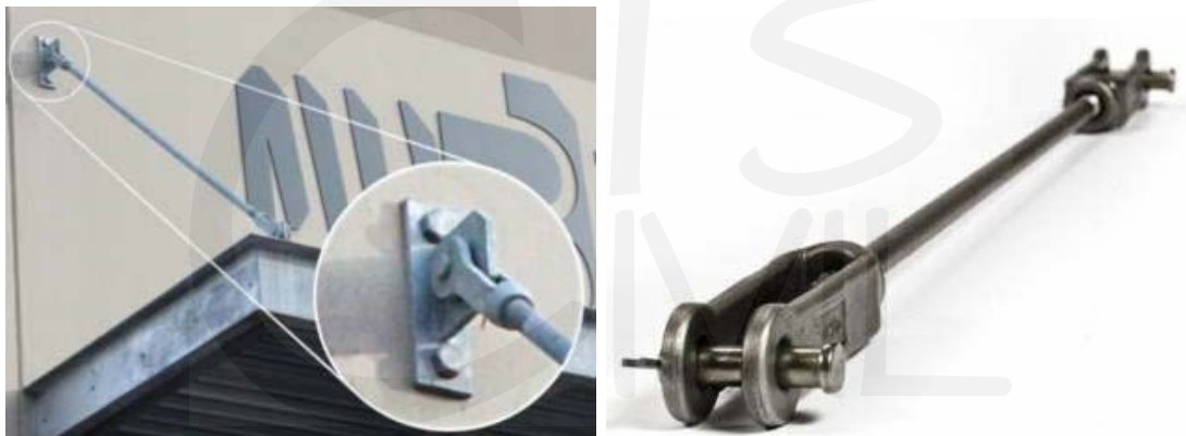
Figure 1-2: Tie Rods
