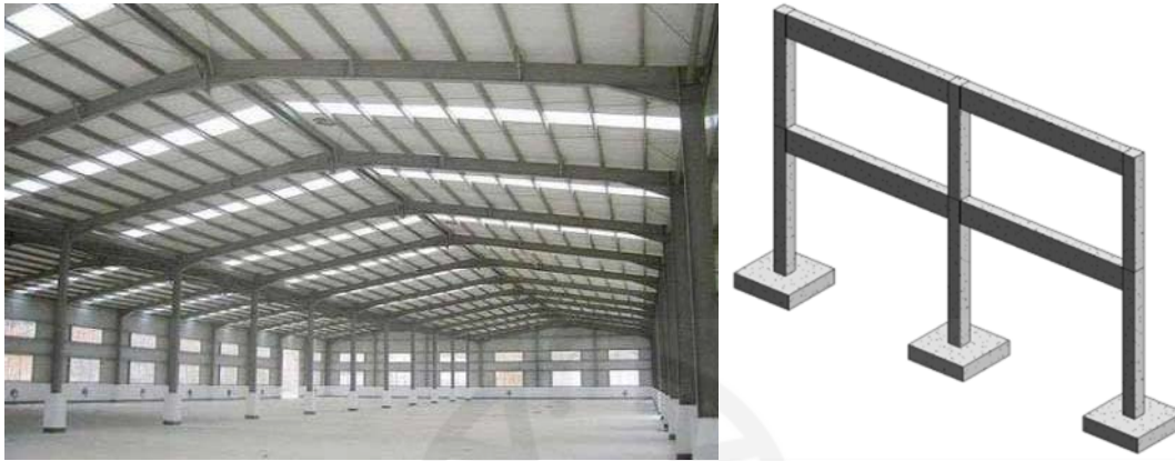
Figure 1-7: Steel and concrete frames
